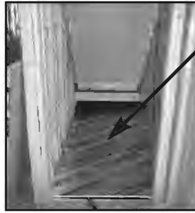
Do not restrict ventilation by blocking openings
