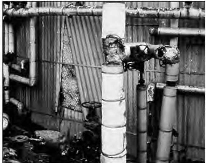
Loose fill insulation
