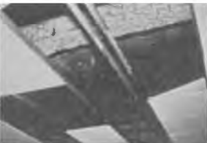
Suspended Ceiling Concealing Fireproofing
