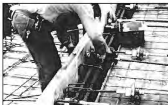
Rodworker attaching anchorage assembly to forms
