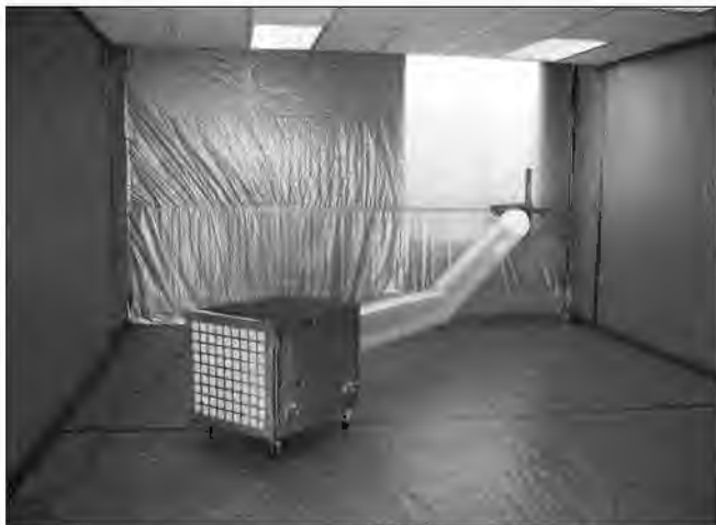
HEPA-filtered negative air unit
