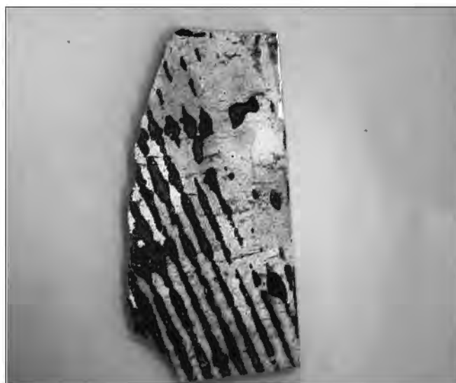
Vinyl asbestos flooring
