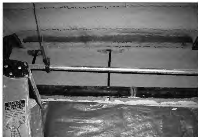
Sprayed-on fireproofing
