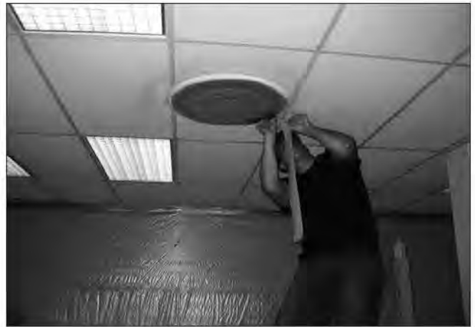
Sealing the ventilation system
