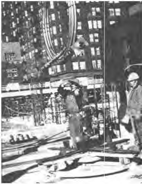
Figure 24 Rigging tendon with nylon slings being lowered on field tendon uncoiler
