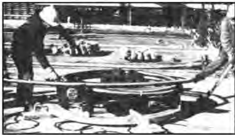
Figure 25 Cutting bands progressively, and crew of rodworkers using the uncoiling turntable
